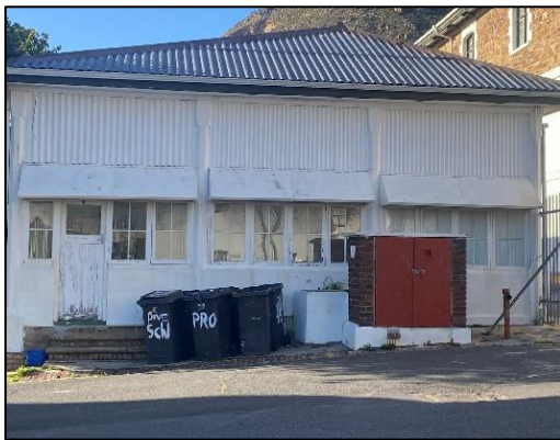
Figure 12. Broken bins standing outside at West Yard.
