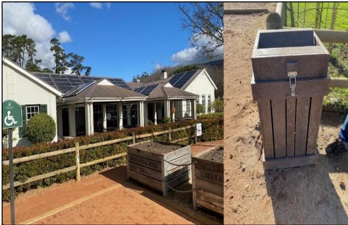
Figure 5. Baboon-proof bins and electric roof apron at Constantia Uitsig.
