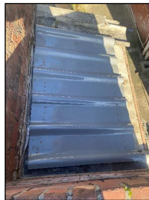
Figure 13. Newly repaired waste room roof at Block R.
