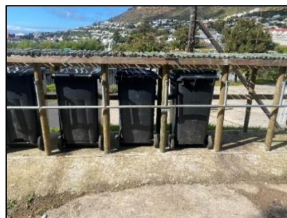
Figure 11. Happy Valley bin storage area.
